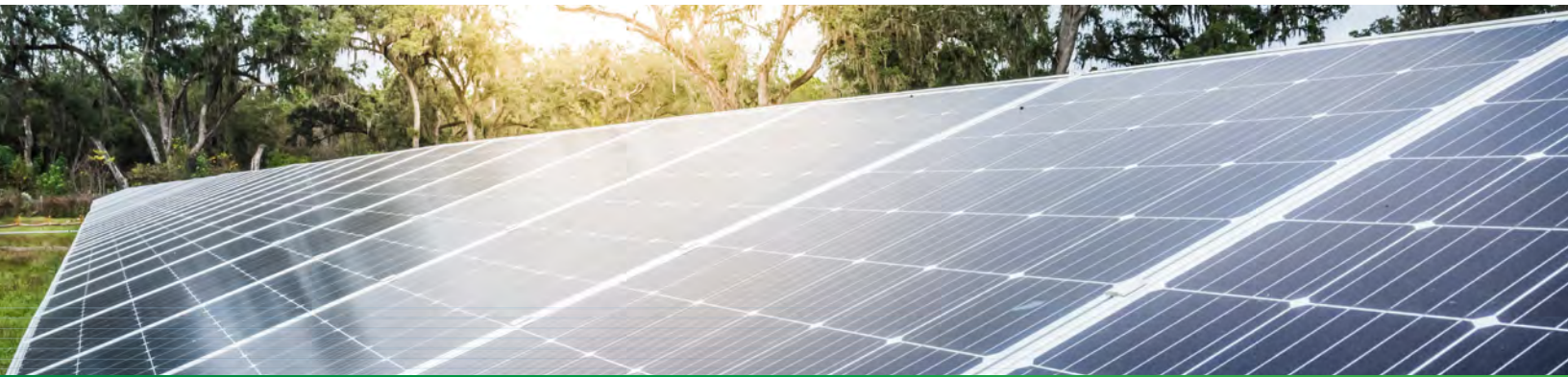
Trenton Solar Facility / Trenton, Florida
