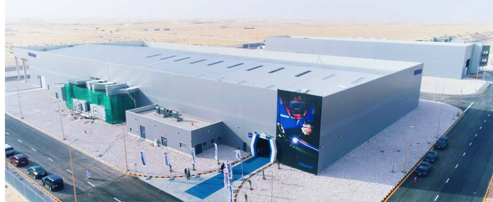
Schlumberger Manufacturing Center opened in 2020 in King Salman Energy Park, Kingdom of Saudi Arabia.
