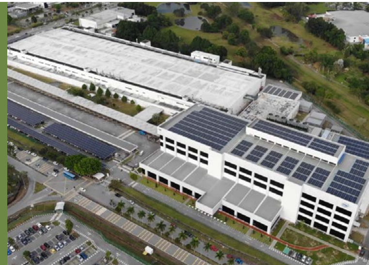
The solar installation at the Intel chip and assembly test manufacturing facility at Kulim Hi Tech Park in Malaysia.
