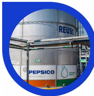
Circular water project at our Sabritas Vallejo plant.
